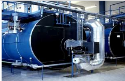
Boiler Water Treatment
